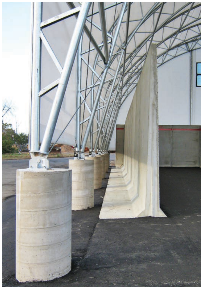
This is an example of Greystone’s design for independent building foundations and pre-cast walls. (Photo provided)
